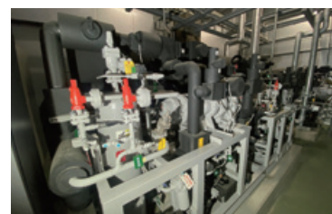
Natural refrigerant system installed at the Jonanjima Refrigerated Warehouse, completed in 2024.
