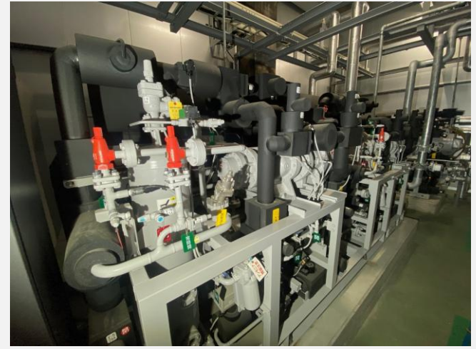
Construction completed in 2024, natural refrigerant equipment at Jonanjima Cold Storage
